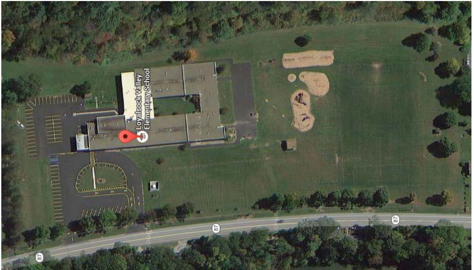
Loyalsock Valley Elementary Existing Site
